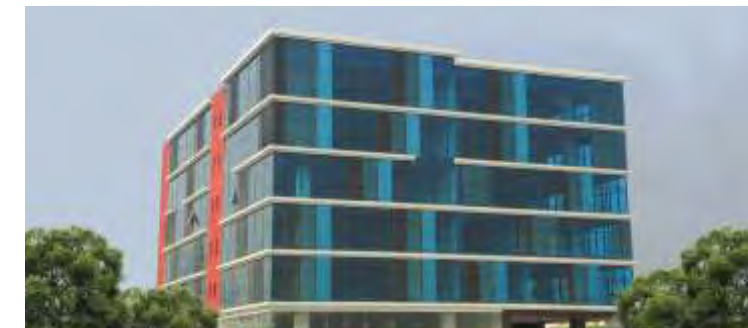
RISHI TECH PARK, New Town, Kolkata (Delivered)
