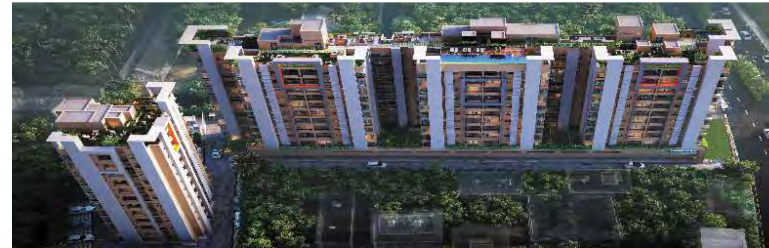
RISHI VENTOSO, Madhyamgram, Kolkata (Under Construction)
